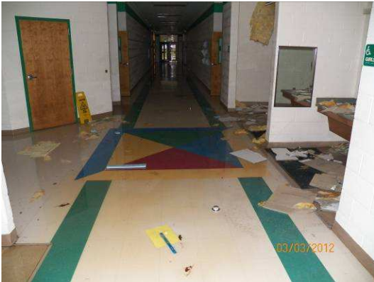
This view shows the main hallway of the wing that suffered the most damage. The areas where students would have been during severe weather were relatively safe with the exception of a few ceiling tiles.
