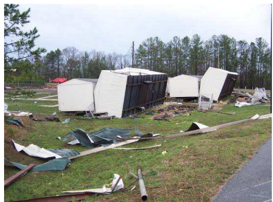
The mobiles damaged were not being used as classrooms.
