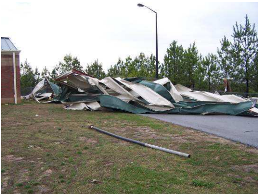
This is the remainder of the roof that was blown from one of the wings. It landed about 50 yards away near another wing of the school.
