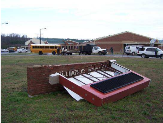
The school's electronic sign was destroyed by the tornado.
