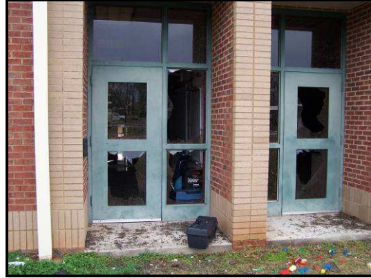
Windows were blown out on several doors and windows at various locations.
