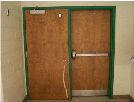
This hallway door was cracked by the power of the F3 tornado.
