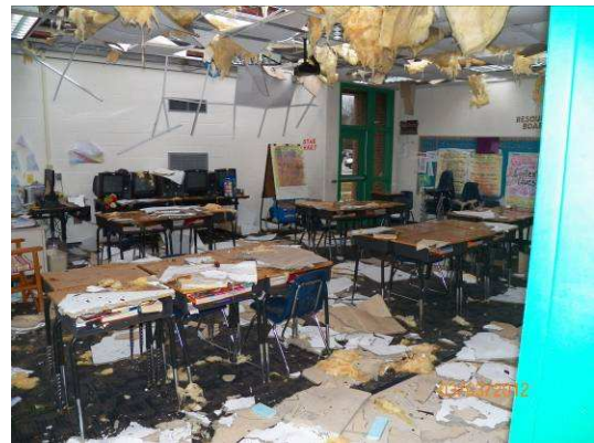
One of the classrooms where the primary roof was blown away
