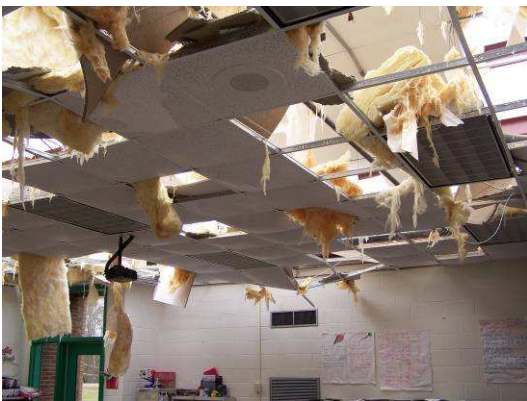
After the tornado hit, heavy rains caused additional damage to the exposed areas.
